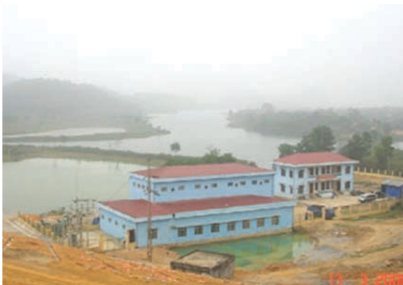
Figure 3.4. Small hydro-electricity plant at Muc River
